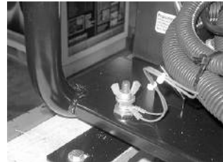
Figure 3-1. Grounding the Generator
